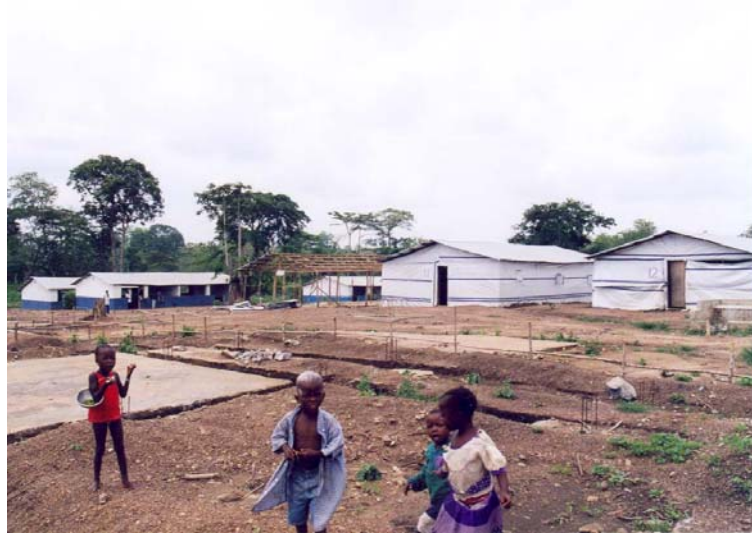
Some of the transit booths, like the ones in the rear of this photo, do find uses after the construction phase, as temporary classrooms or storage areas. But their structures are not stable, and more of them are collapsing as the storms of the rainy season approach. Image: Kennedy
